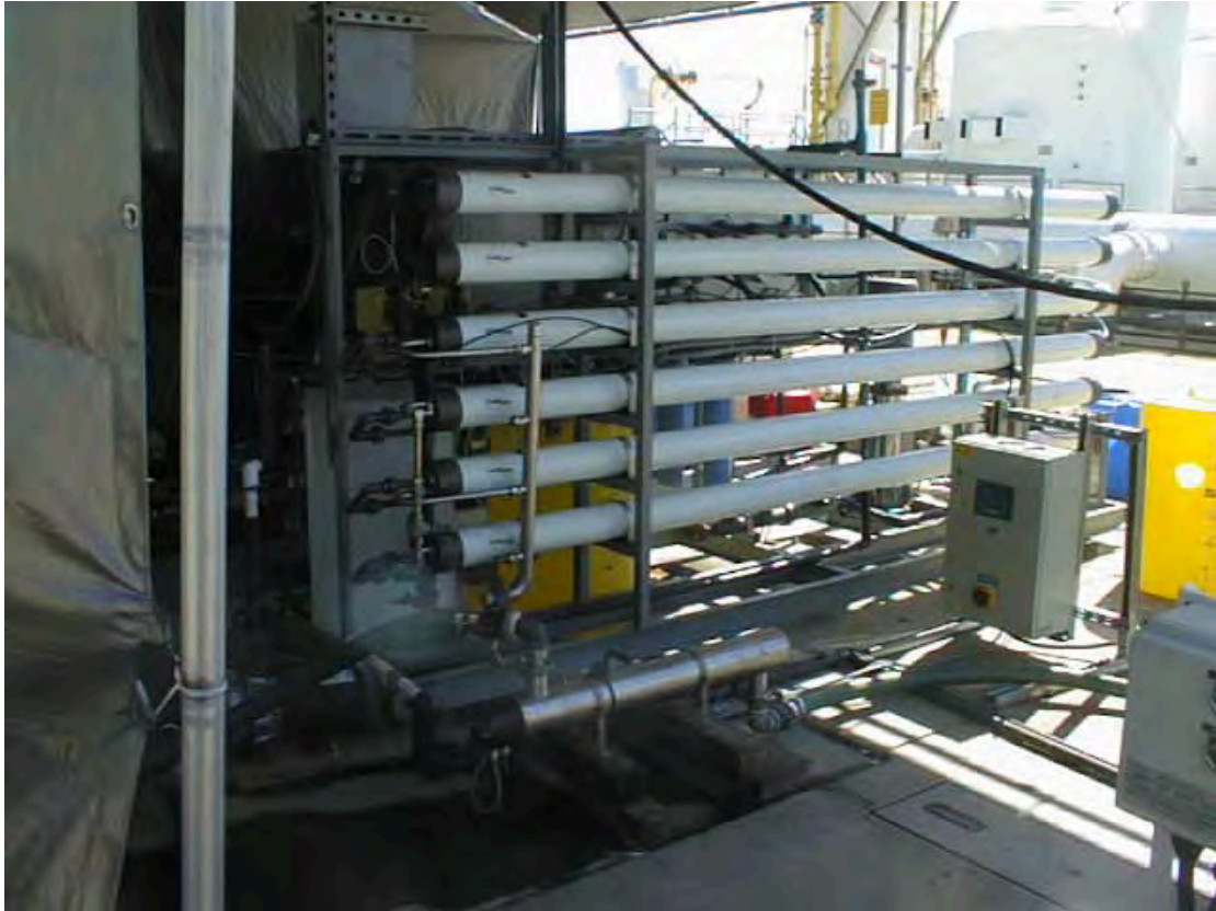
RO Pilot Skid
