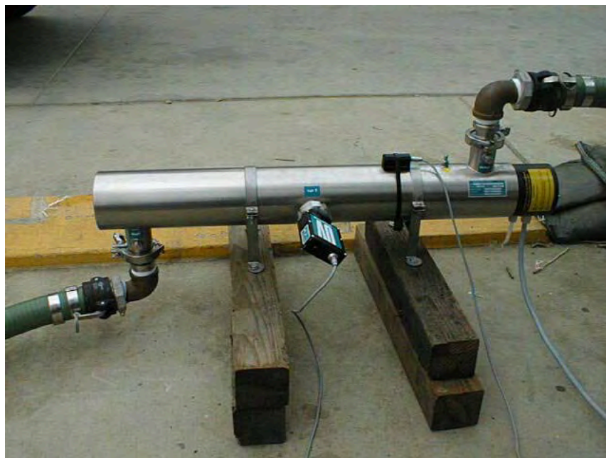
Aquionics UV Pilot System – Control Panel (Top); UV Reactor (Bottom)
